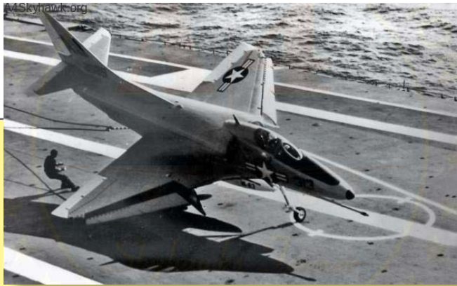
A bad day! A-4C 148589 of VA-83 on 17 May 1963. The Skyhawk was susceptible to tipping up on a wing. U.S. Navy photo.
